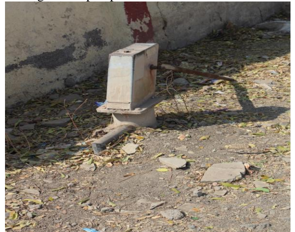
Fig. 10 Damaged Handpump
