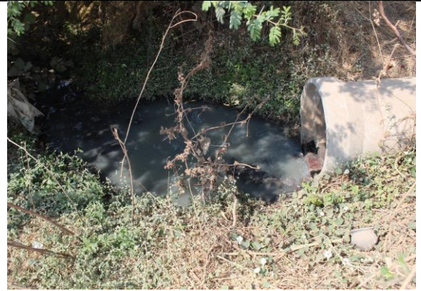
Fig. 9 Outlet of sewer
