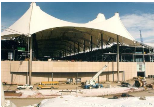
Figure 1- Tensile membrane structure.
