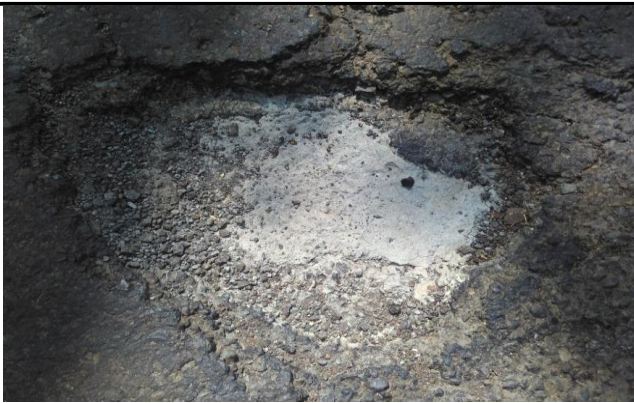
Figure no. 7: Actual pothole filled
