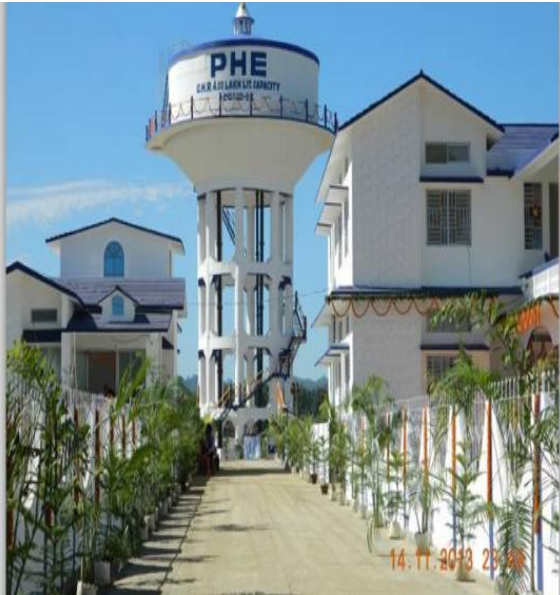
Fig.3 ELEVATED SERVICE RESERVOIR IN PUBLIC HEALTH ENGINEERING DEPARTMENT
