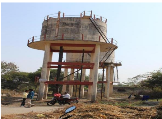
Fig.4 CIRCULAR TYPE ELEVATED SERVICE RESERVOIR
