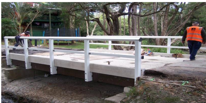
Fig. 1- GPC Deck type bridge
