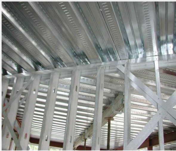
Fig10. Light Gauge Steel Structure
