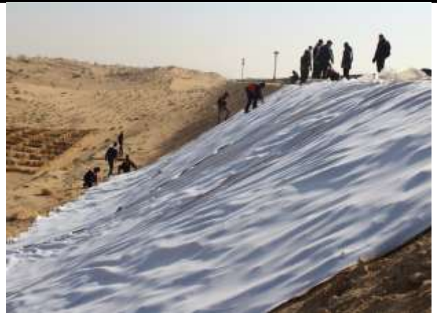
Figure-1. The process of laying geotextile on the slopes of the subgrade (Kiyikli – Khizirbobo stage km 4199 PK 1)
