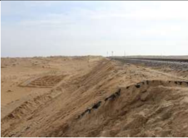
Figure-4. Final view of strengthening the slopes of the roadbed with geosynthetic materials (Kiyikli-Khizirbobo stage km 4199 PK 1)
