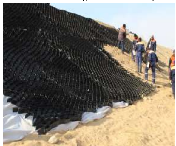
Figure-3. The process of filling the geogrid cells with local soil with parallel sowing of sand-loving grass seeds (Kiyikli – Khizirbobo stage km 4199 PK 1)
