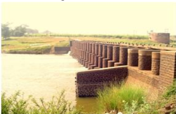
Fig. 18 Check dam site.
