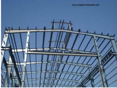
Fig 2. Site Construction work of PEB structure.
