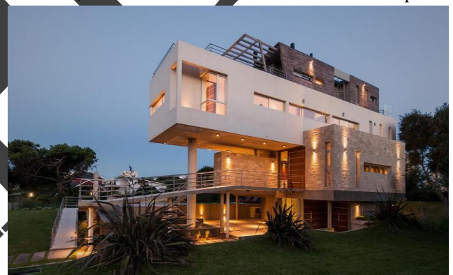
Fig 1.1: Hotel building having floating column
