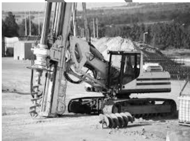
Fig. No. 7: Earthmoving machinery
