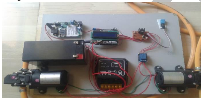
Hardware of Automatic control
