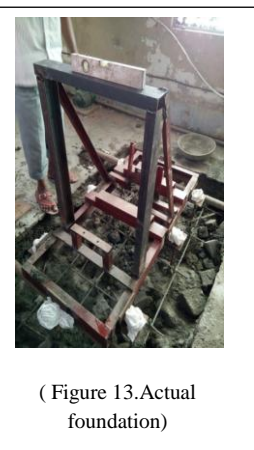
( Figure 12. Arrangements for foundation bolts )
