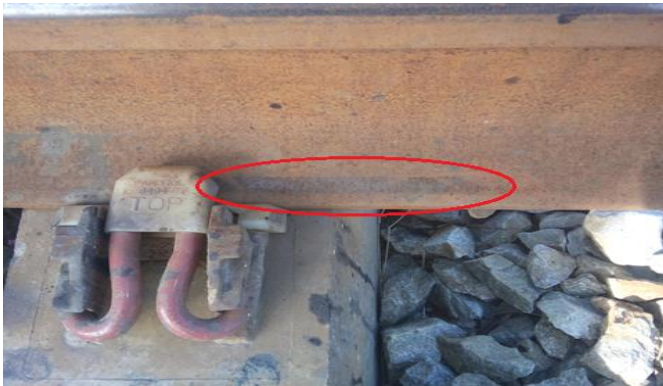
Figure 1. Traces of the terminal on the sole of the rail at the longitudinal displacement of the lashes.
