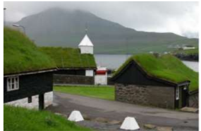
Fig-1. Houses with green roofs in the Faroe Islands.
