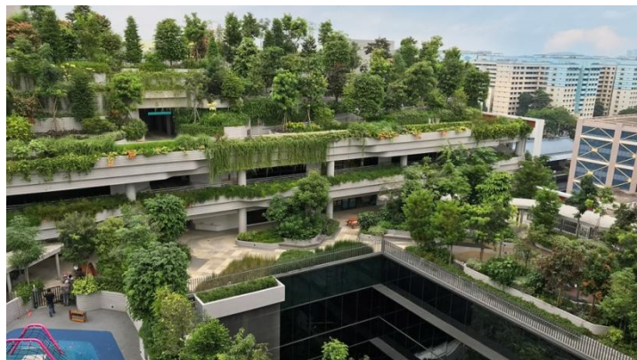
Figure 10. An example of Green Roof Gardens in Singapore
