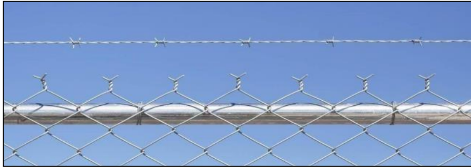
Figure 3: Wire Differences in Chain-Link Fences
