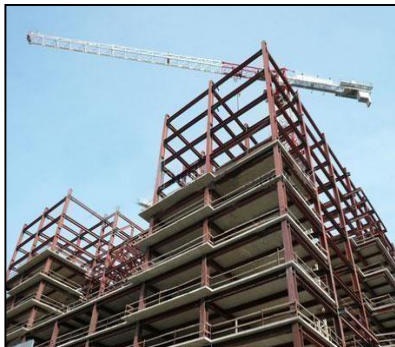
Typical composite structure
