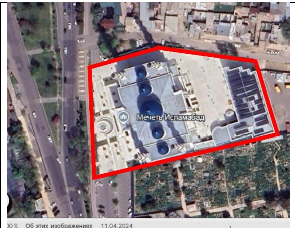
Figure 3. Islamabad Mosque Current Status.
