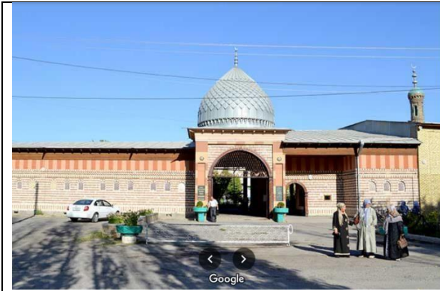
Figure 4. Islamabad mosque in its former state.
