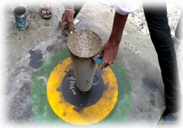
Fig 9 Working method with slump cone
